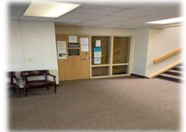
Office Suite 130 Entrance
